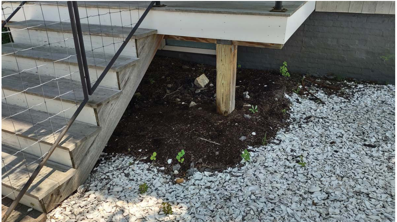
Entry porch posts in contact with wet soil.
