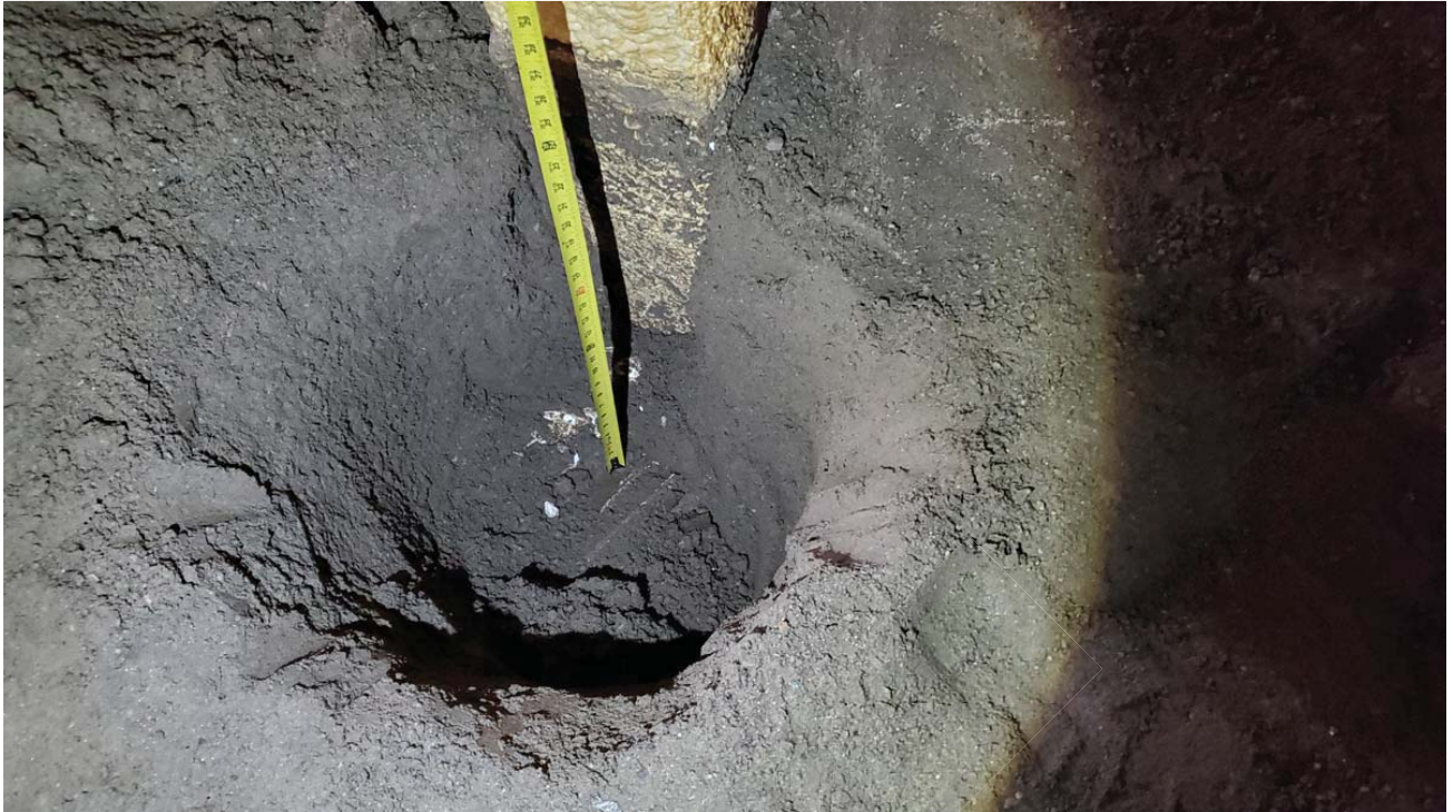
Excavation at the columns reveals 2' to the bottom of the original column. Spray applied insulation was wet below grade.
