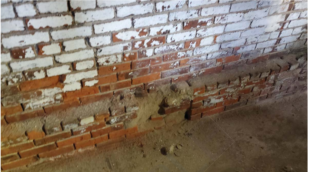
Interior of Utility Building foundation has extensive deterioration to the brick and mortar.
