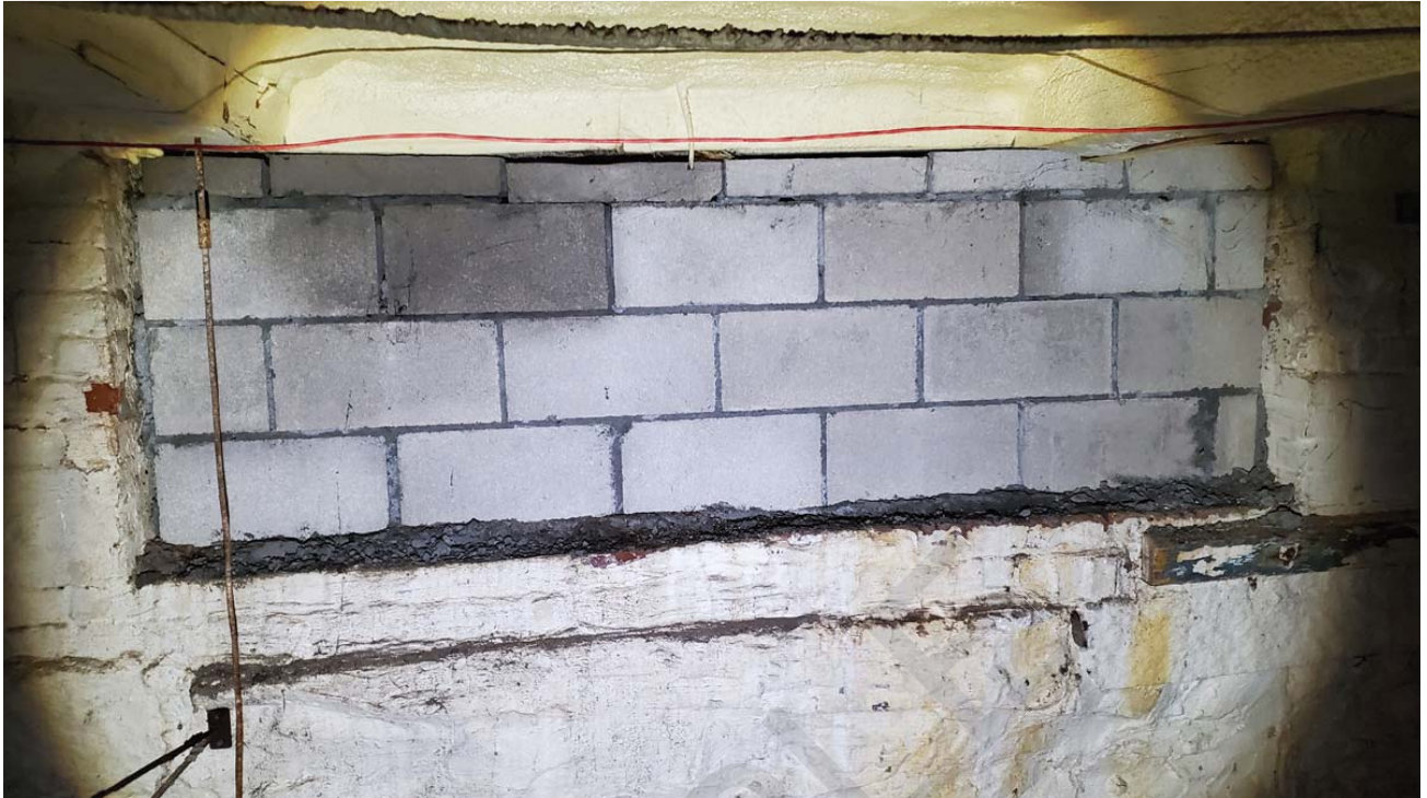
An added section of concrete block does not properly support the sill.
