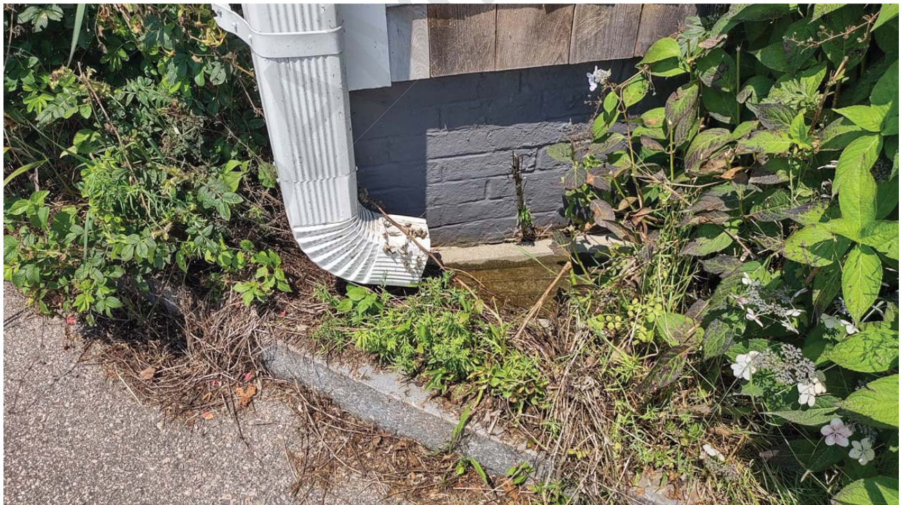
Poor roof drainage and downspouts lead runoff water directly to the foundation.
