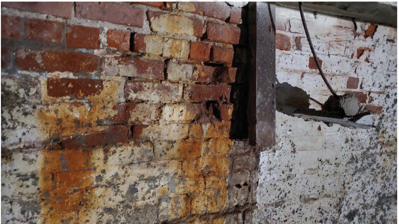
Some areas of the upper brick foundation walls were bulged inward due to soil pressure against deteriorated brickwork.
