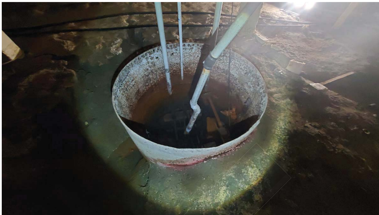
Sump pit receives drain water from above. Pump abandoned and non-functioning.
