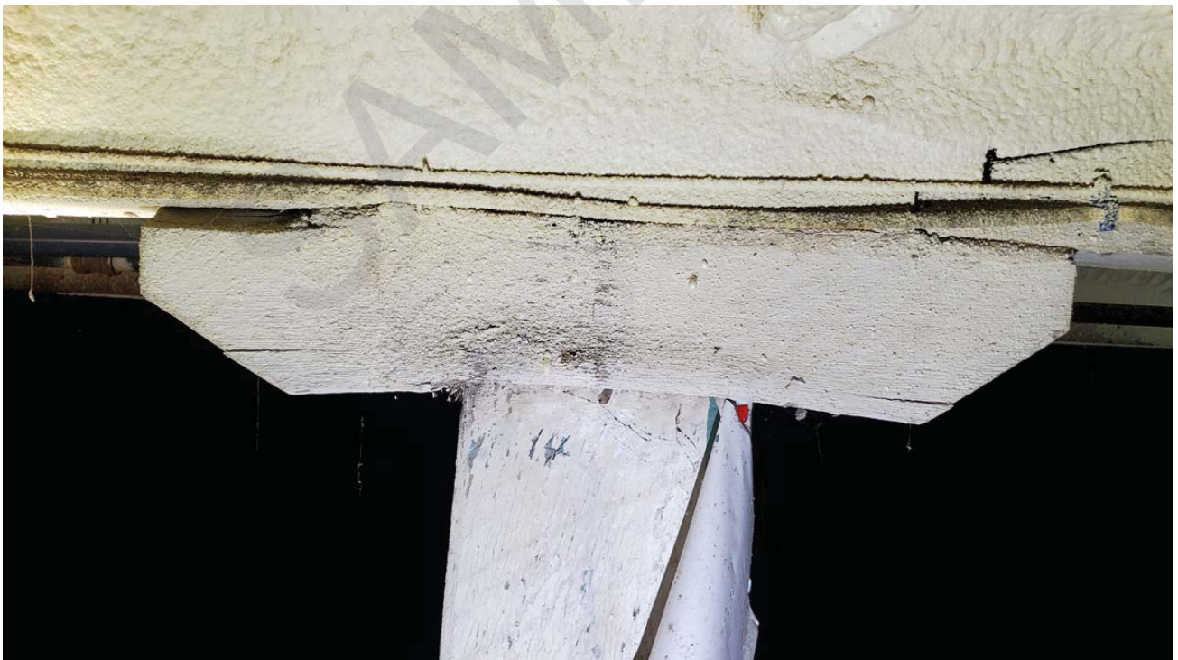
Other haunches were severely deformed due to compressive loads.
