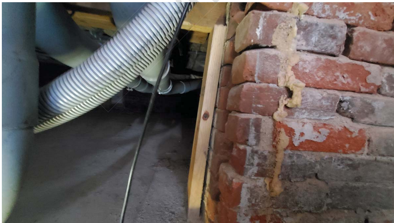
Utility building floor system inadequately supported by 2x4 post.
