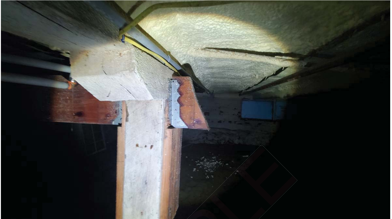
Wood haunches atop the timber columns were cracked in some locations.
