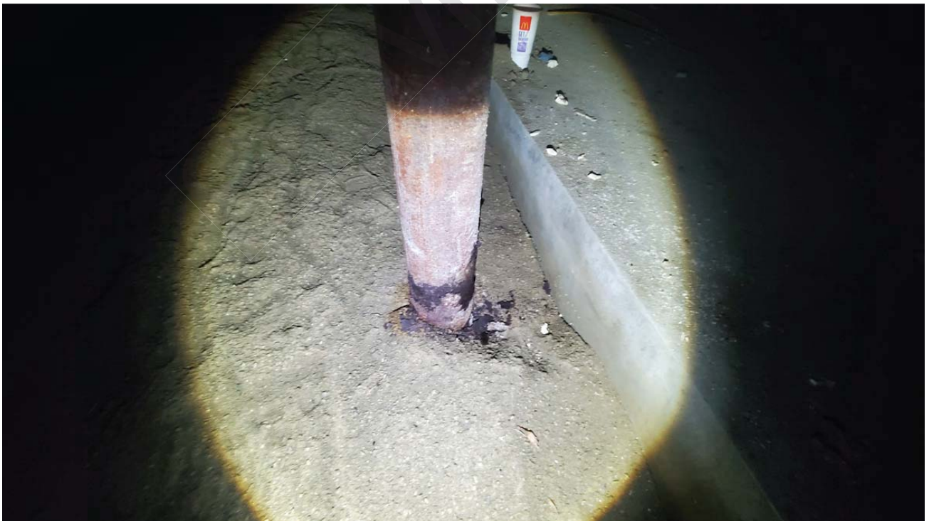
Steel column is corroding due to its contact with damp soil.
